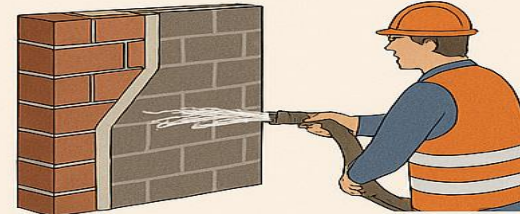
Installing Insulation in Existing Buildings
