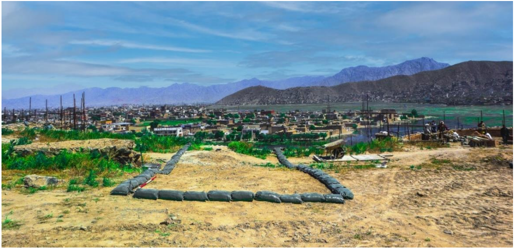
Figure 15: General view of trench 10 th , before excavation zone 2 (photo by: AKTC_A).
